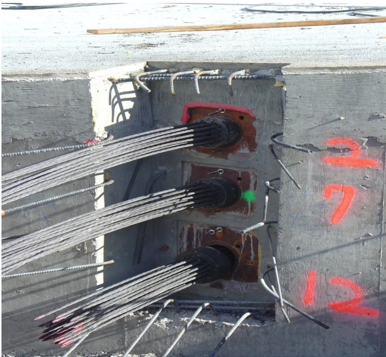
Fig -40 Post-tensioning on a highway overpass
