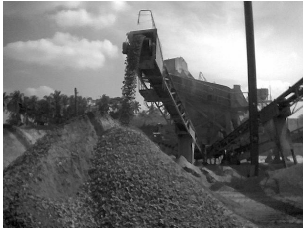
Fig -6 AGGREGATE BASE COURSE AT CRUSHER PLANT
