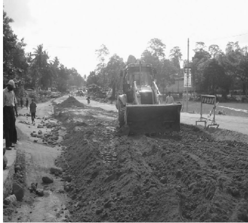
Fig -4Sub Base Constructions
