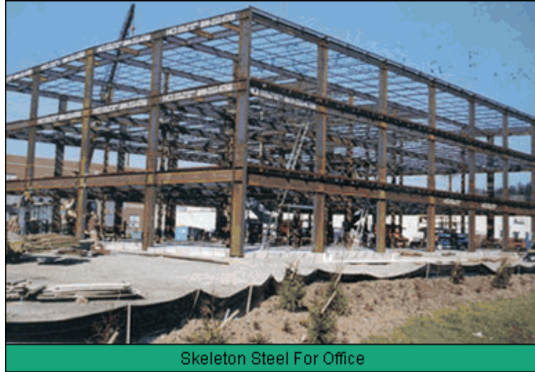
Fig : 18 A STEEL STRUCTURE
