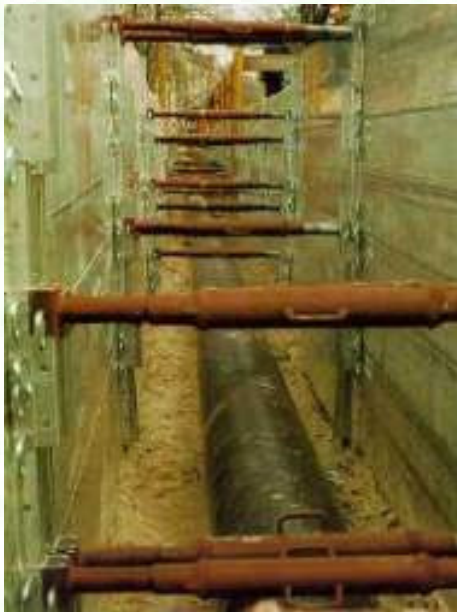
Example of shoring and a trench box
