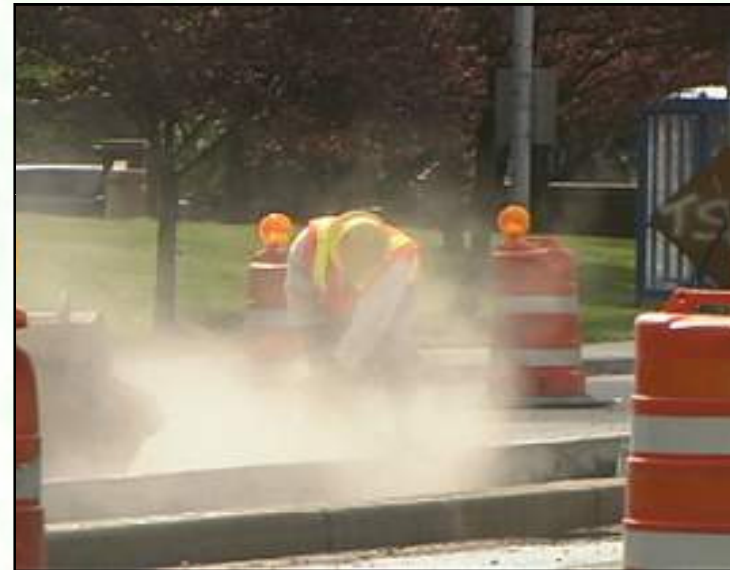
Silica exposure from cutting concrete in road construction
