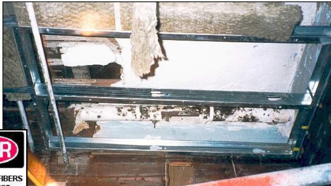
Damaged asbestos pipe insulation ©CSC Campus
